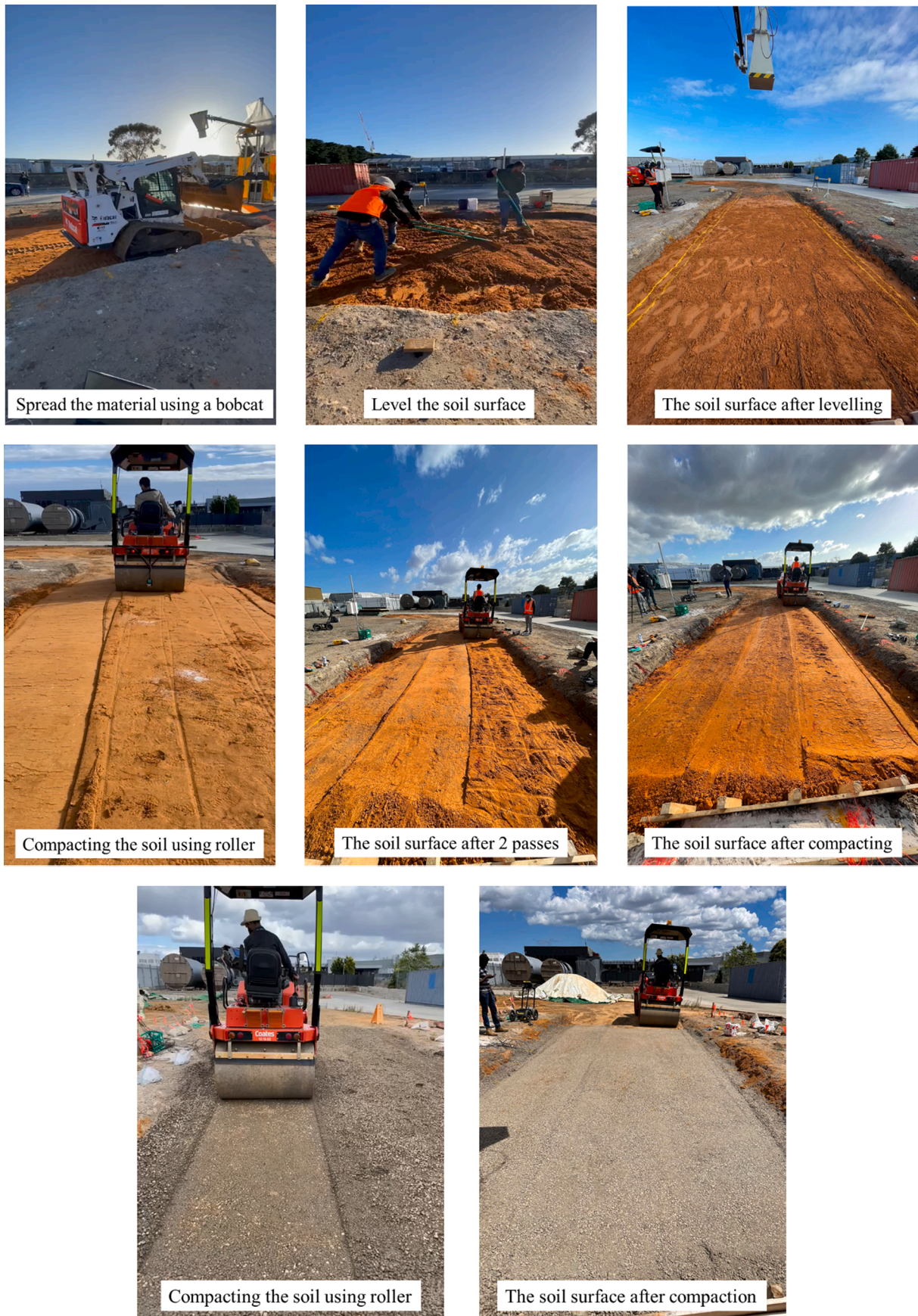
Fig. 5. The compaction process consisted of evenly spreading the transported material to the test-bed using a bobcat, levelling the surface and conducting compaction with a roller for sand subgrade (from left to right, top to middle). The procedures for UGM sub base/base were similar and are shown in the two images at the bottom.
