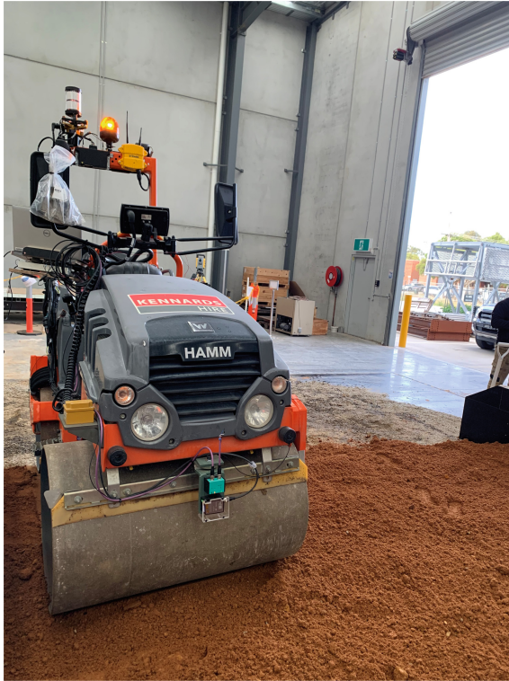
Fig. 3. Picture of Instrumented roller before compaction
