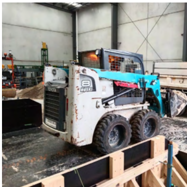
(a) Placing the material using a bobcat
