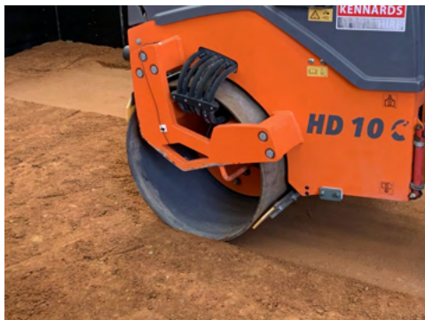
(c) Compacting the material using the instrumented roller
