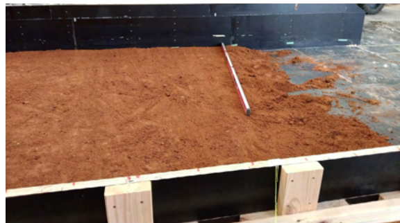
(b) Spreading the material manually using shovels and rakes and levelling using a bubble level
