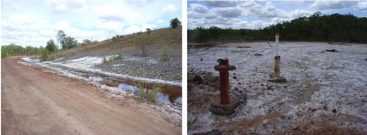
Figure 6. Rehabilitation of waste rock, Rum Jungle, July 2007, ~25 years after rehabilitation : (left) White’s waste rock dump and acid mine drainage, (right) adjacent East Finnis River during the dry season (no flow) showing the cumulative effects of acid mine drainage. (photos – author)
