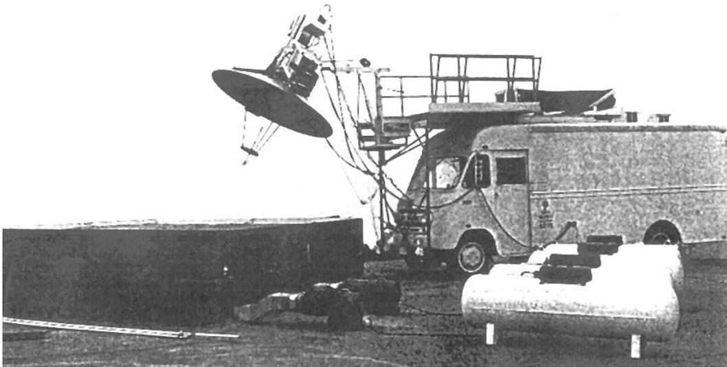
Figure 2.6: An example of a ground-based system. The system comprises a "truck"-mounted radiometer, making observations of a sand target area. Data processing equipment is contained within the van (Njoku and Kong, 1977).
