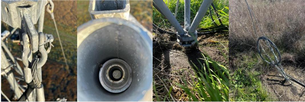
Figure 2: Bow shackle, Ladsaf spring, Mast base, Guy point of the tower
