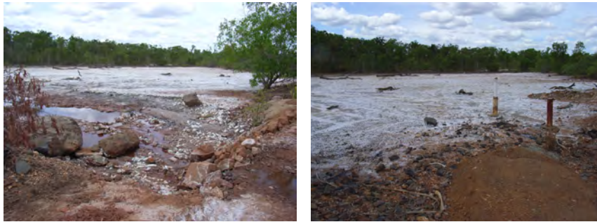
Fig.7. Former Sweetwater Dam, July 2007; Note – the water and flow in the left photo is continuing seepage from White’s waste rock dump (see Fig. 3) (photo's G M Mudd).
